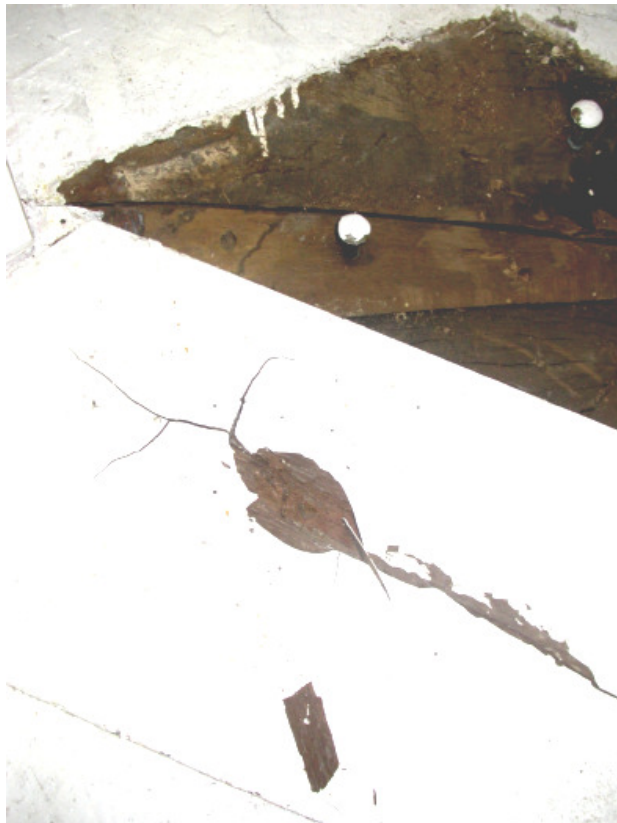
Fig 11: Decay in the painted planks
