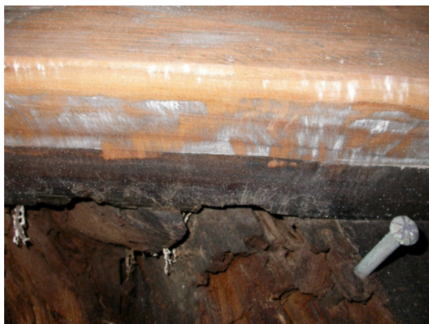
Fig 5 (left): Deteriorated rafter in the back
