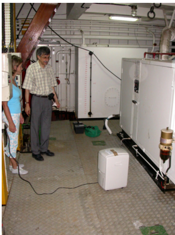
Fig. 9: condensation air-dryer in the technical room in the middle of the vessel.
